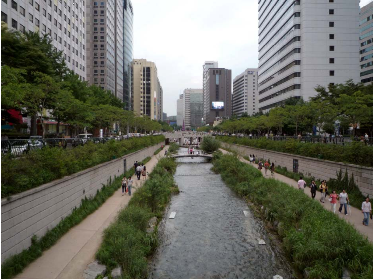
Fig. 4: With the demolition of a multi-lane, multi-storey highway which was built in the 1960s, the Cheonggye river was transformed into a popular recreation area. The core element is a new, artificial river crossing the center of the city of Seoul. The promenades along the river are used by a large number of citizens. © Hea-Jee Im.
