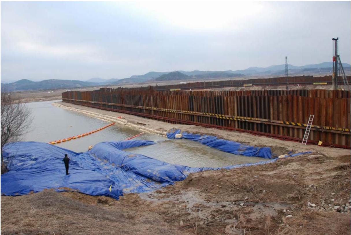
Fig. 2: Construction site of the Buyeo barrage on the Geum river. The Buyeo barrage is 7 m high and 620 m long (500 m is stationary and mounted and 120 m is maneuverable). The retention volume is 23.5 million cubic meters. After completion, the average river depth will be 4.6 m, the average width 294 m. © Byoung-Sung Choi
