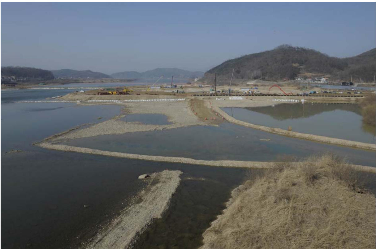
Fig. 2: Construction site of the Buyeo barrage on the Geum river. The Buyeo barrage is 7 m high and 620 m long (500 m is stationary and mounted and 120 m is maneuverable). The retention volume is 23.5 million cubic meters. After completion, the average river depth will be 4.6 m, the average width 294 m. © Byoung-Sung Choi
